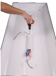
The metal enclosure of driver must be grounded.
